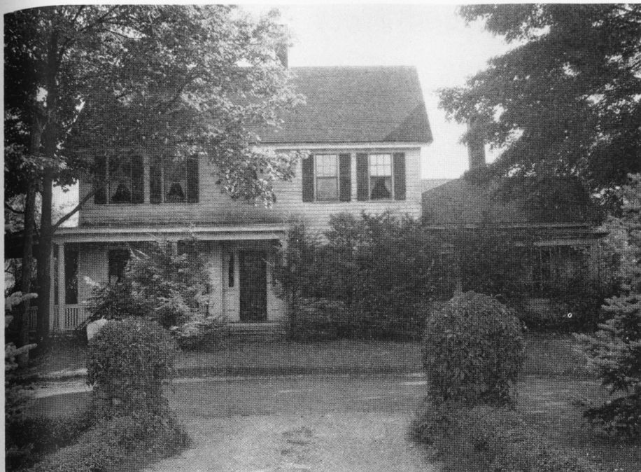
This is the beautiful old Cornelis house on the Scovill property out near Woodtick. It can readily be seen how easily this fine old home could be remodeled so as to serve as a general recreation headquarters for all SERA activities centered in the area.
